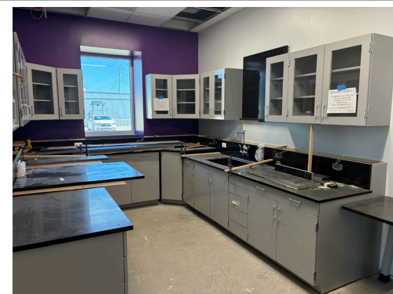
Other work on the project recently includes the installation of cabinets and counter tops in the lab room.
