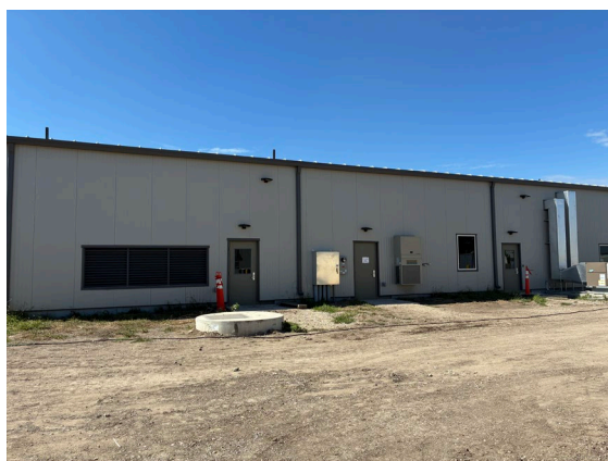
East face of the new plant building.
