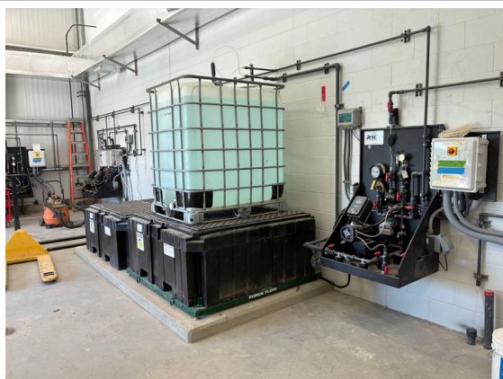
The installation of chemical feed skids and spill containment devices in the chemical room had been taking place.
